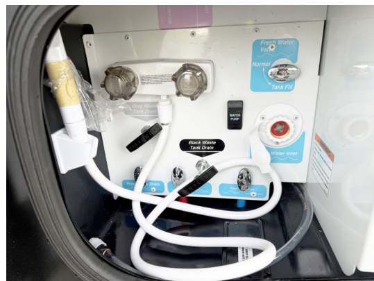
Exterior Shower/Wash Station (524D) -Typical View
