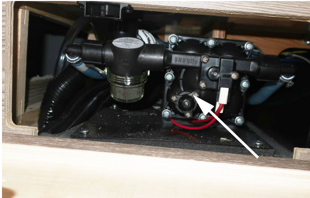
Water Pump (Access Panel snaps back on.) -Model 524T shown -Typical View
